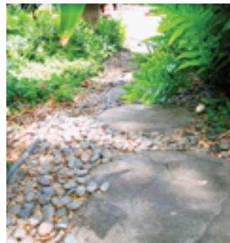
This paving option uses impervious pavers; however, space is left between each paver (and filled with gravel or grass), thus allowing water to pass through and get absorbed. ‘Stepping stones’ are an example of semi-permeable paving.
