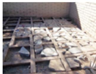
This is a semi-permeable option that pieces together fragments of concrete slabs (available free from construction or demolition job sites) in creative ways. The spaces in between the slabs allows for permeability.
