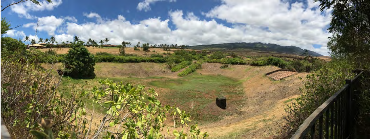
Figure 18: Example of an off-stream retention/infiltration basin. High flows from the stream enter the basin, and sediment settles out as water infiltrates into the ground. Overflows are failsafe mechanisms necessary if the basin becomes overwhelmed by excessive stormwater. The access road at the far side of the basin allows for periodic removal of sediment with heavy equipment.
