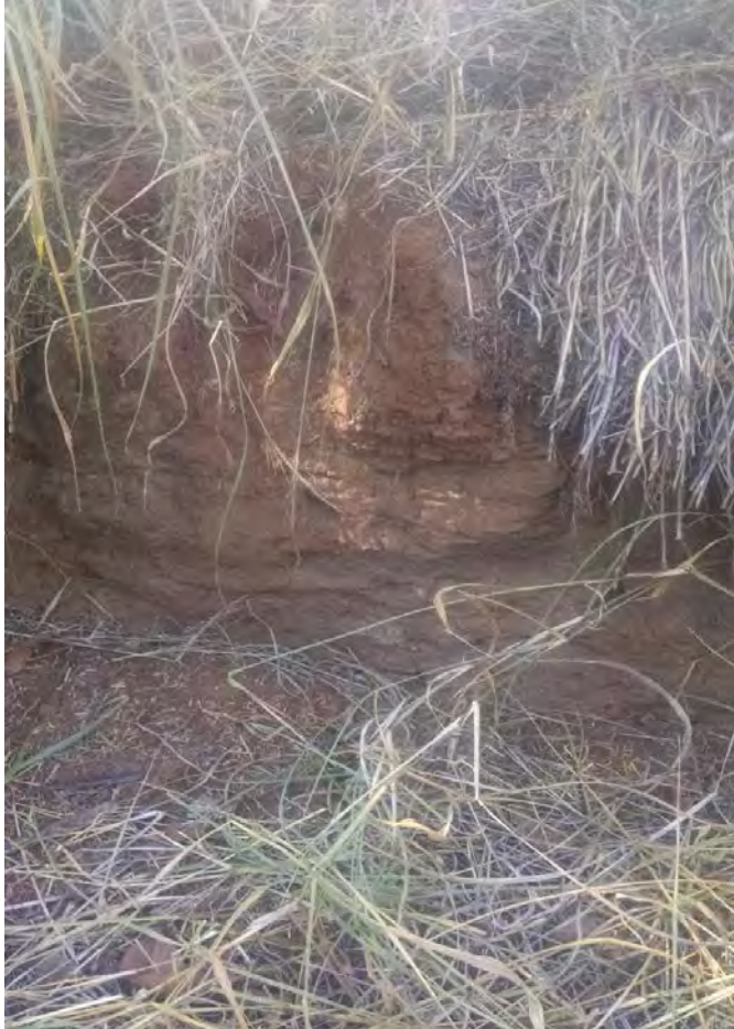
Figure 17: Test pit showing overburden of fine clay (approximately 3-5 feet thick). This layer would have to be breached in order to effectively utilize infiltration wells or trenches.
