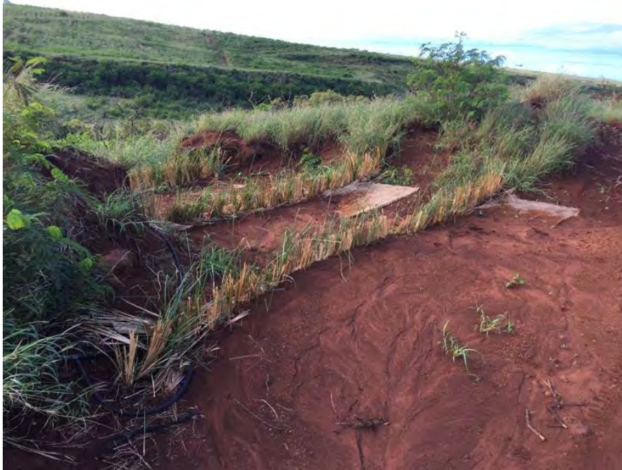
Figure 6: Vetiver half-moon pilots planted in a road kickout in Wahikuli under Ridge to Reefs' NFWF grant. This photo was taken one month after installation and already shows significant volumes of sediment retention.
