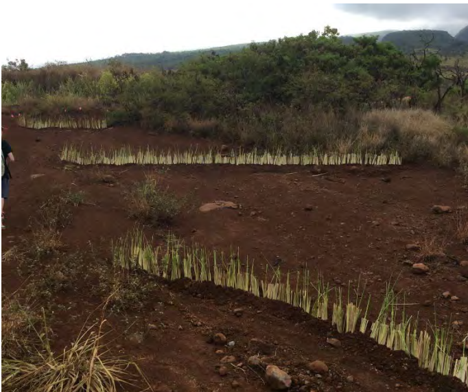
Figure 8: Example of vetiver planted on contour for hillslope stabilization following spacing slope and guidelines outlined in NRCS practice 601.
